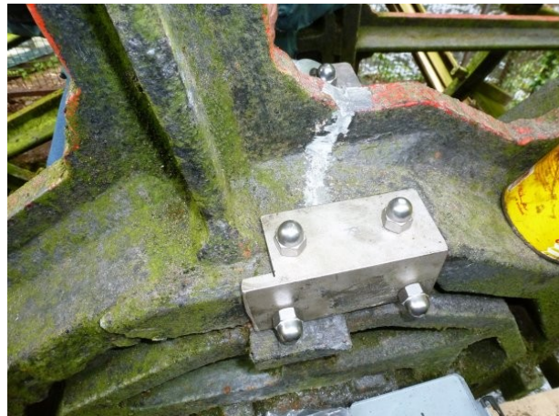
The repair completed on 30th June 2016.
