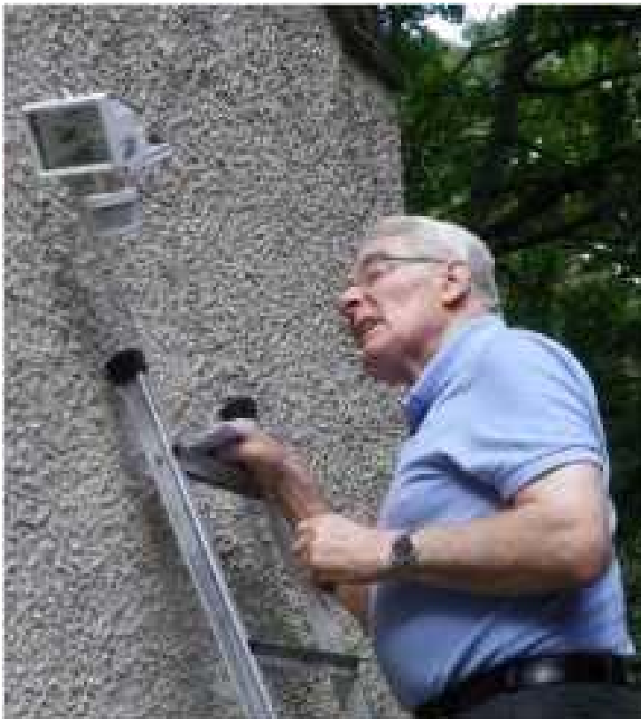
Figure 4 Eric at work on the security light (photo M. Taylor)
