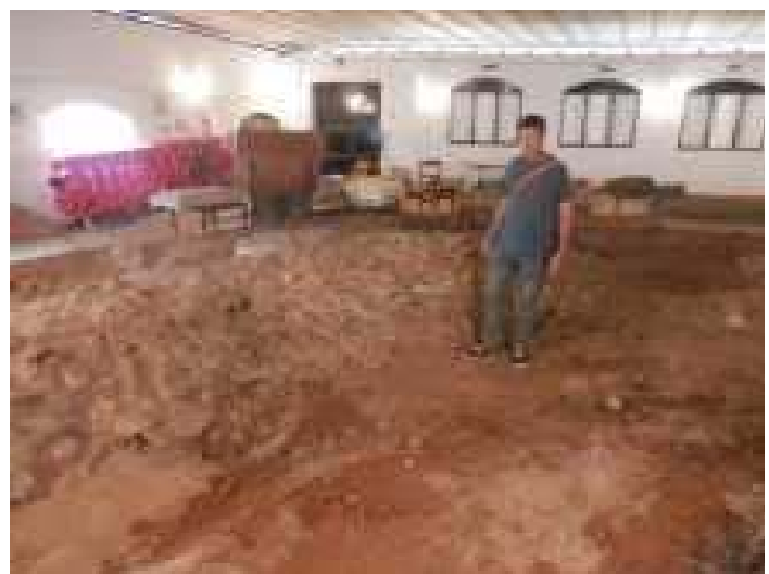
Figure 6 Dave Saxby giving some idea of how high these walls now are.
