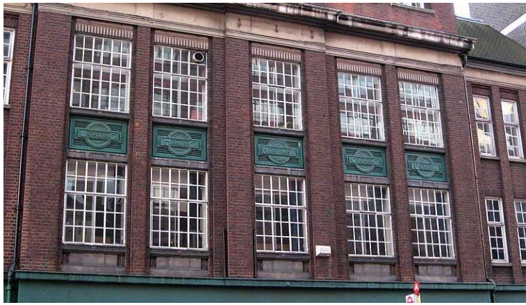
Figure 12: The Northmet building. Photo courtesy the website (see text)
